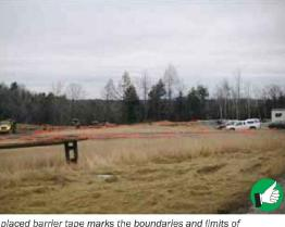
Properly placed barrier tape marks the boundaries and limits of construction on this site.
